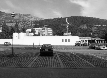
Figure 6 Outside view on the Slovenian Beach seawater heat pump assisted system.
