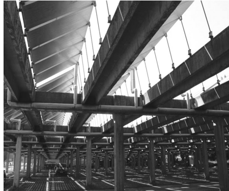
Figure 3 Slovenian Beach—Seawater heat pump assisted solar system's flat plate collector field.
