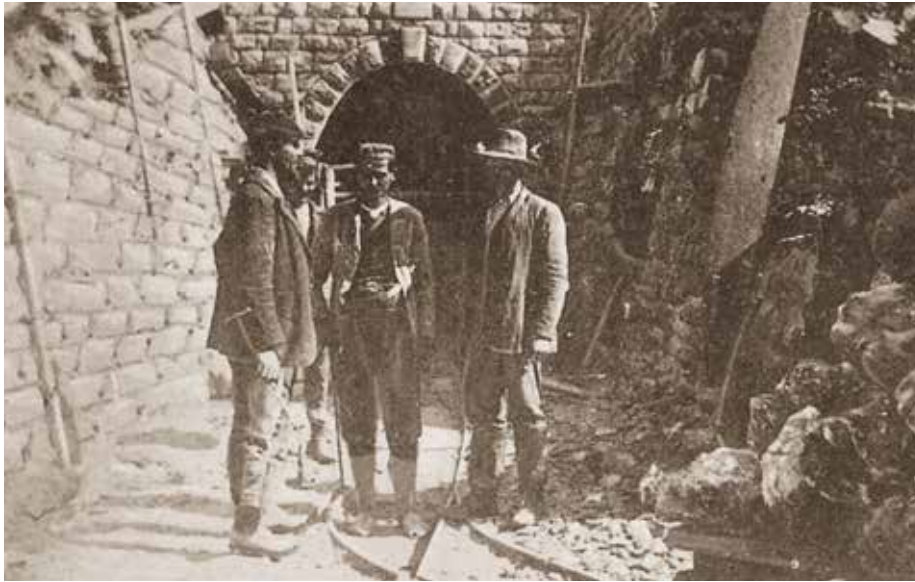
Radovi na probijanju tunela Sutorman, foto: https://dd-shaz.blogspot.com/2017
