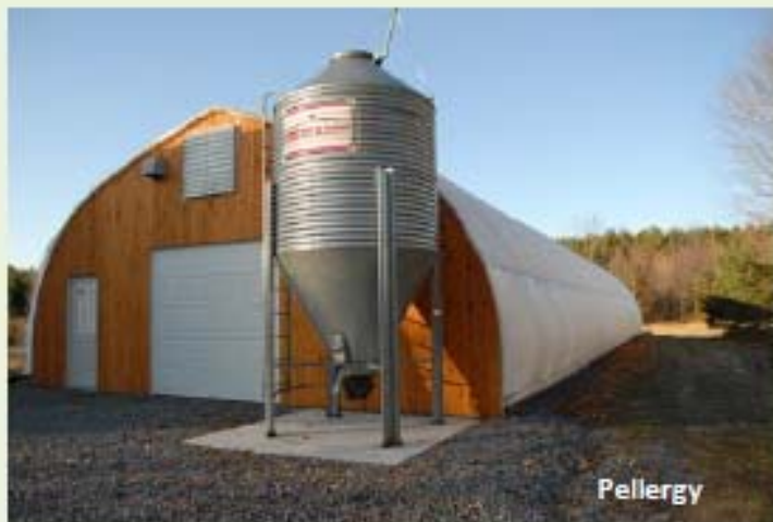
Figure 15, Selected internal and external pellet storage options
