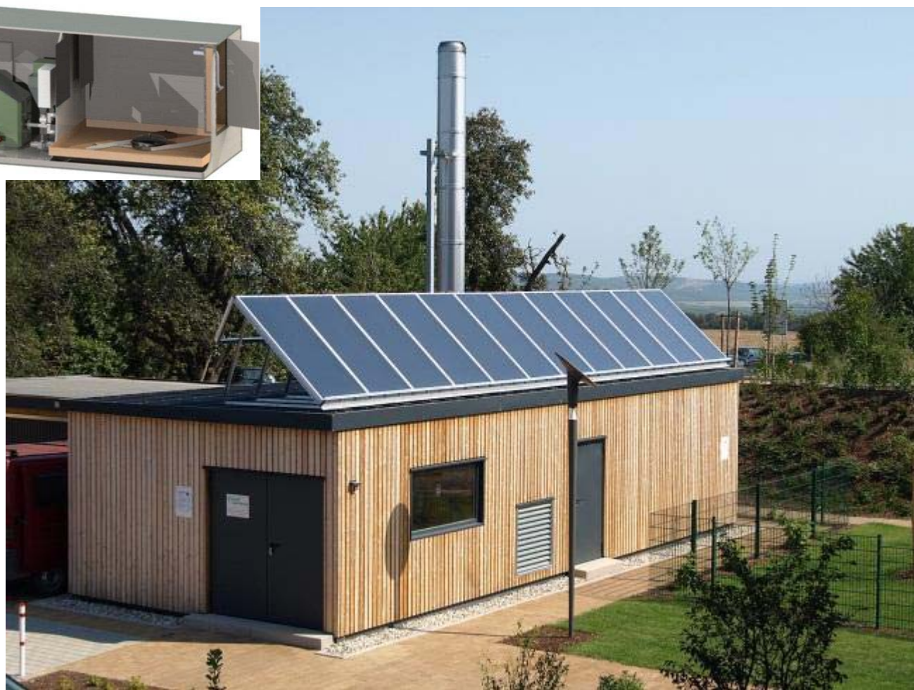
Containerised biomass heating cabins
