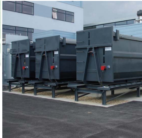
Figure 16, Automatic ash extraction auger from stepped grate boiler and external ash bin
