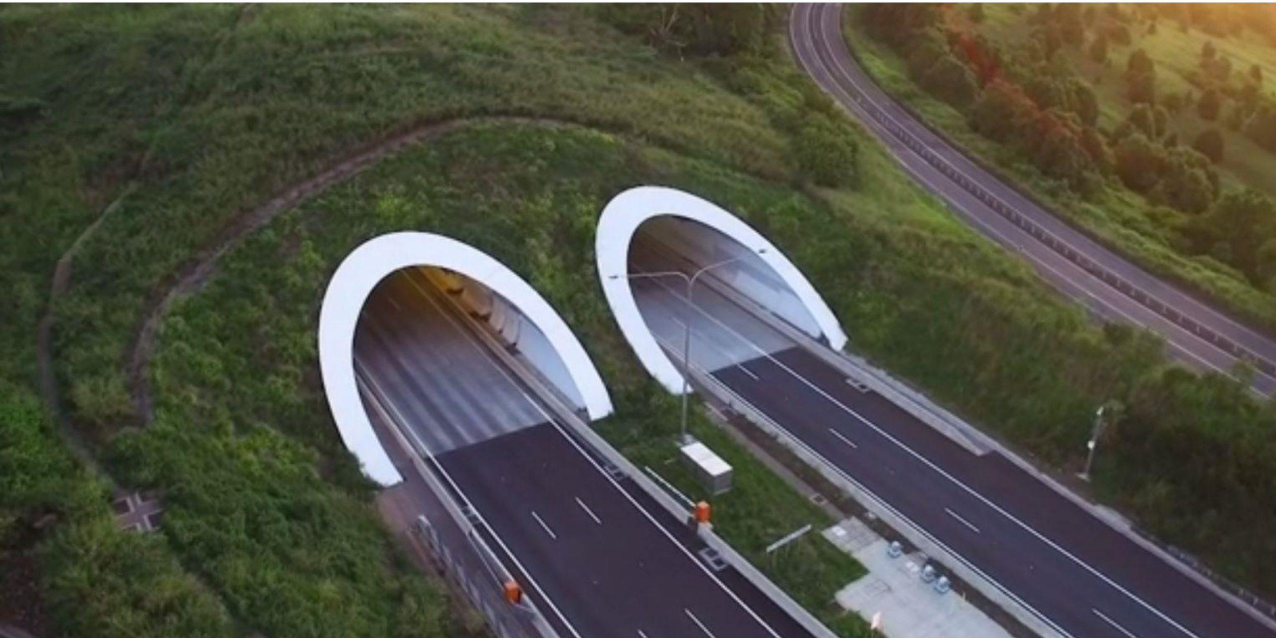
St Helena tunnel, Pacific coast highway, SAD
