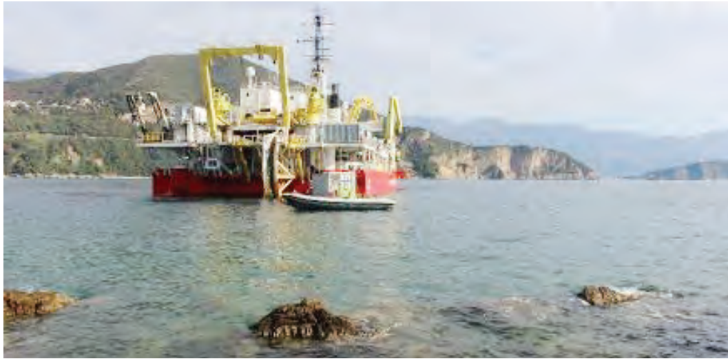
Figure 5: phase of submarine cable laying (Montenegrin side)
